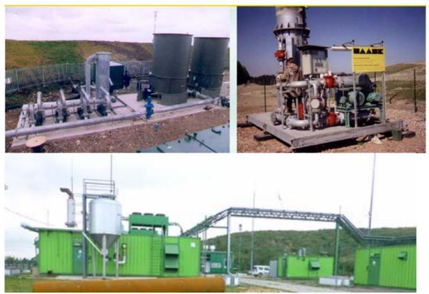
Figure 7 – Booster and flares system (top) booster and CHP units (above)
