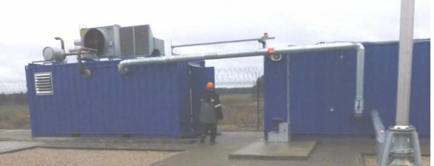
Figure 8 Containerised booster system and gensets (CHP units) Clarke Energy Ltd. in Wales (top) and Vireo in Belarus (below)
