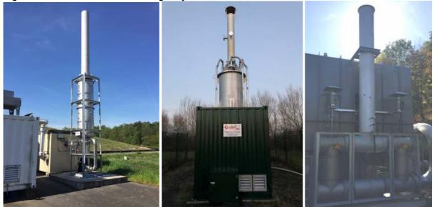
Figure 12 – Low calorific flares right > 12 Vol % CH<sub>4</sub>, middle > 5 Vol % CH<sub>4</sub>, left < 5 Vol % CH<sub>4</sub>
