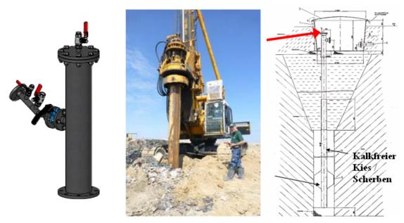
Figure 2 – Landfill gas wells (head) / drilling / complete gas well
